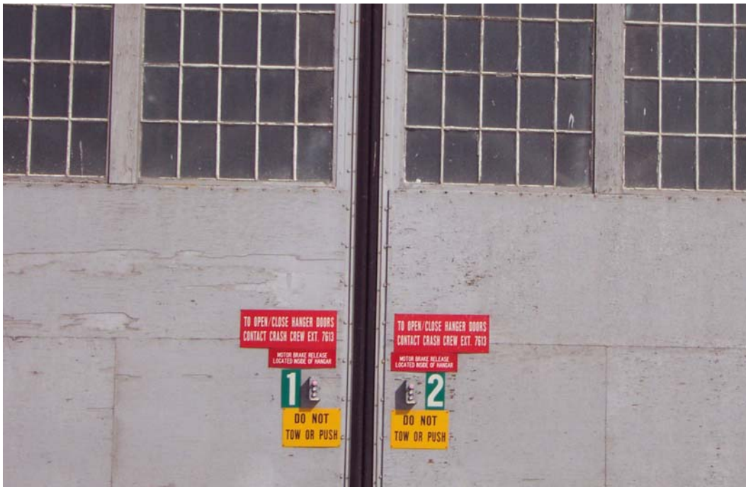
Building 28 exterior, south door detail, March 2002
