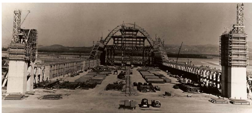
Hangar under construction, 1942
