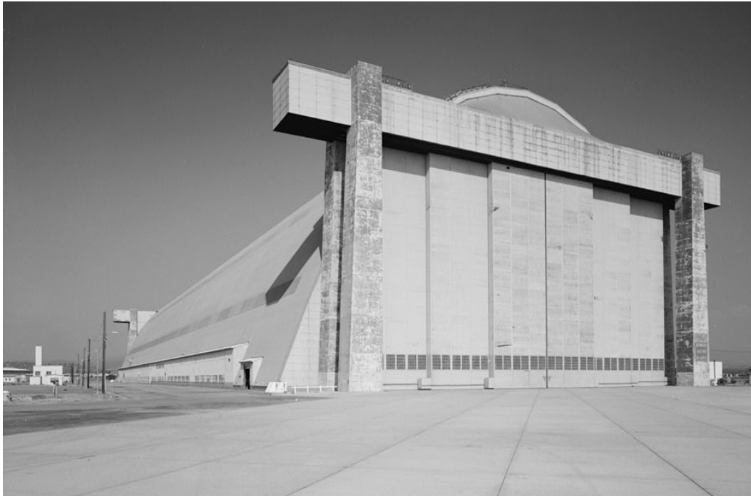
Building 28 (Hangar 1), south doors, 1999
