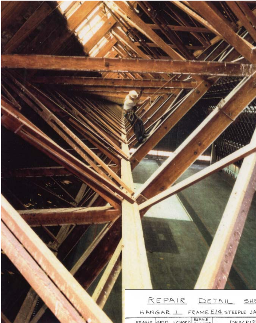
A civilian steeplejack inspects a portion of a roof truss, 1997.
