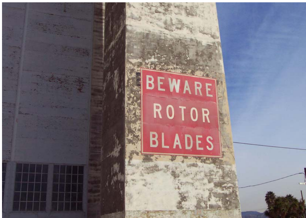
Warning sign, Building 28, March 2002
