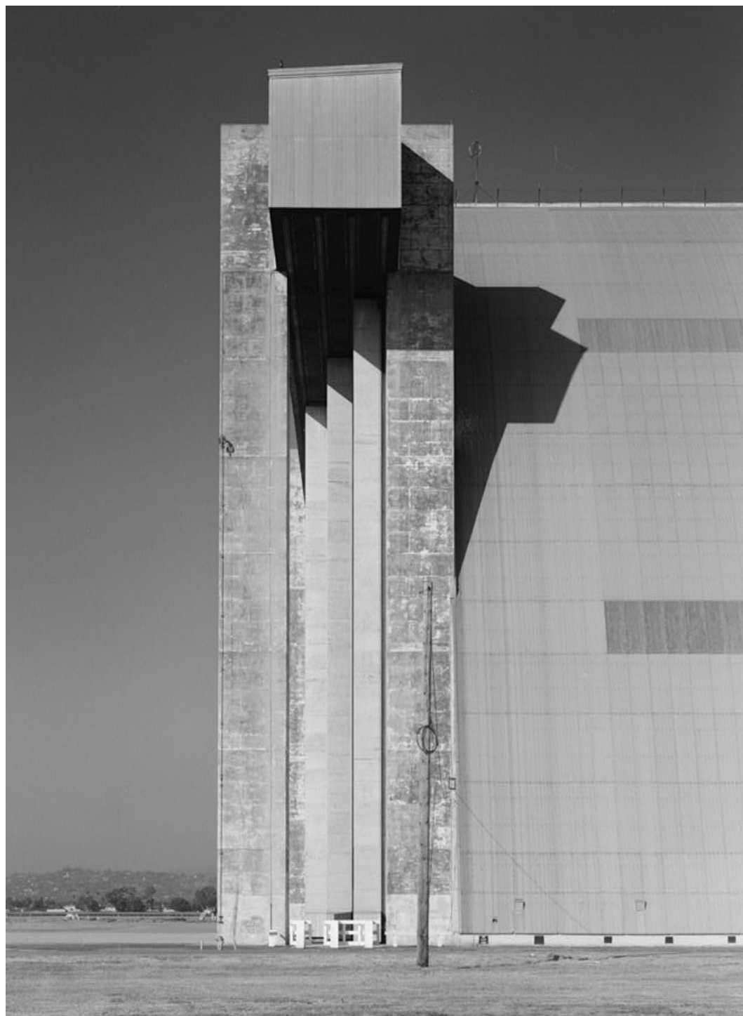
Building 29, west doors, 1999
