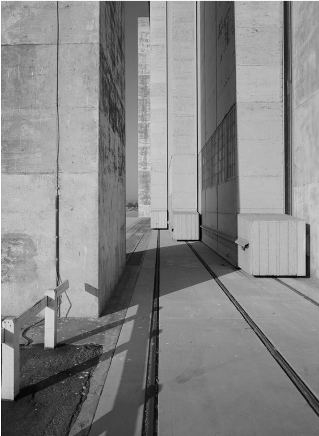
Building 29, west doors, on rails, 1999
