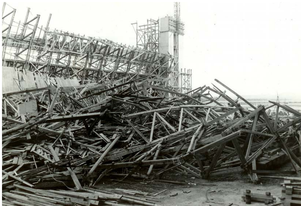
Building 29 following windstorm collapse, January 23, 1943
