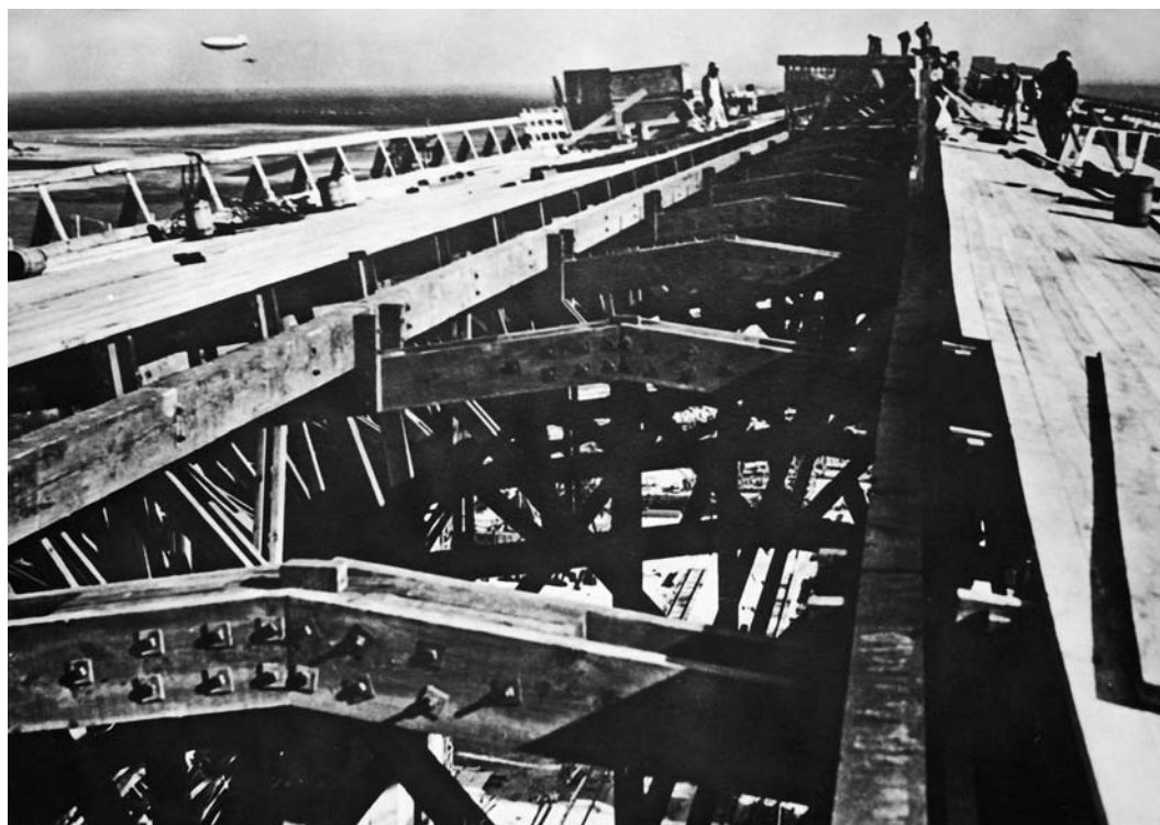
Hangar roof under construction, 1942, USN blimp in flight, upper left
