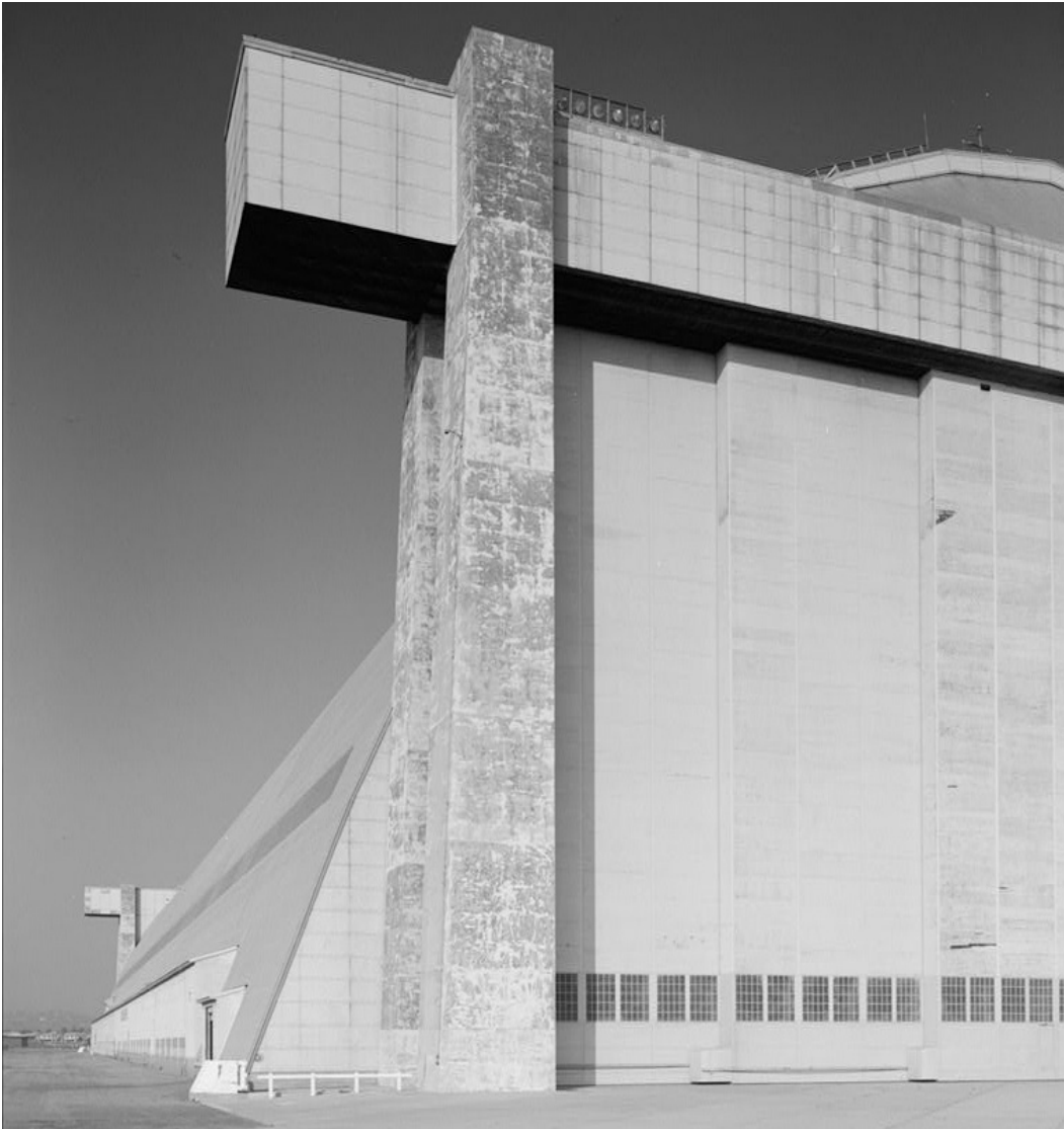
Building 28, north doors, 1999
