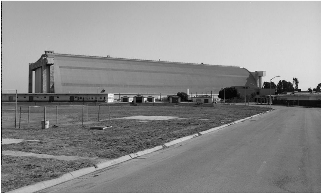
Building 28, west side, 1999
