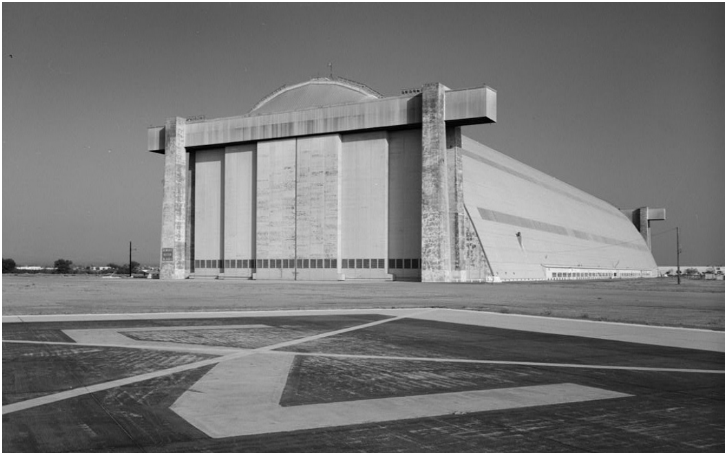
Building 29, west doors, 1999
