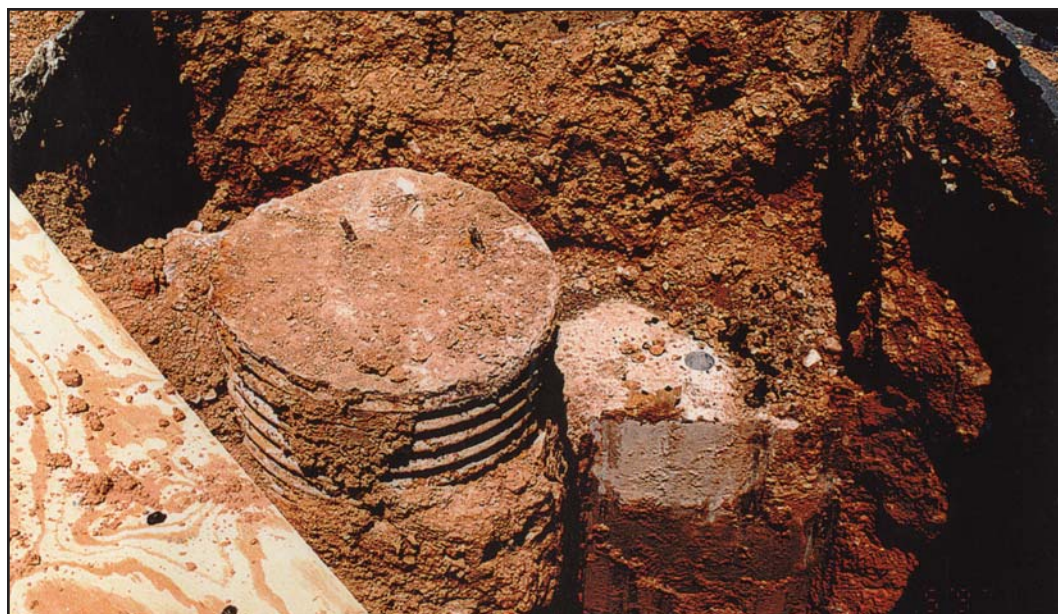
One of the 1,600 Raymond piles beneath the hangar foundations exposed during a 1997 inspection.
