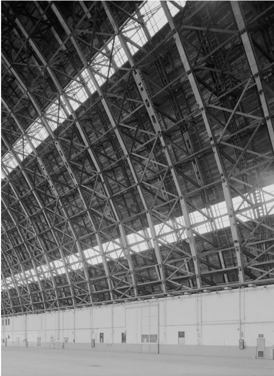
Building 28, wall-roof detail, 1999
