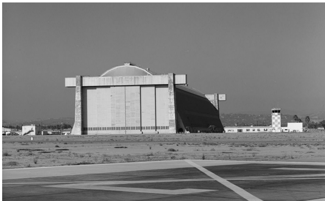
Building 28, south view, control tower on right, 1999
