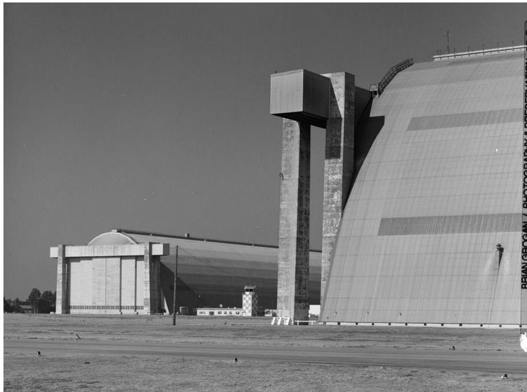
Building 29, right, Building 28 in background, 1999
