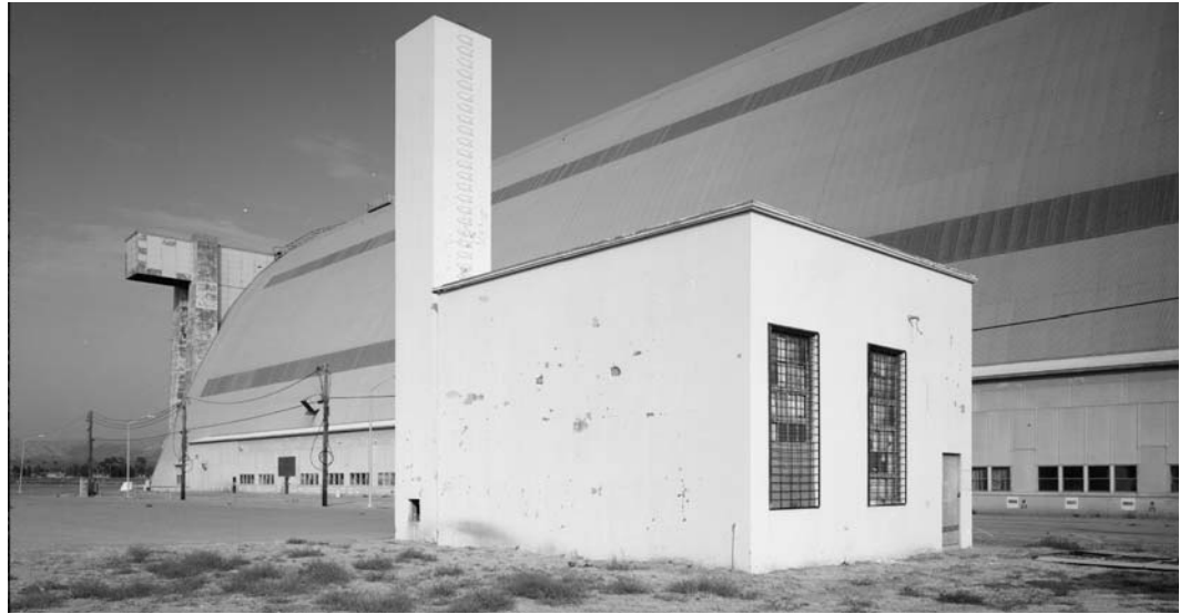
Helium Tank Building No. 1 (Building 28A)
